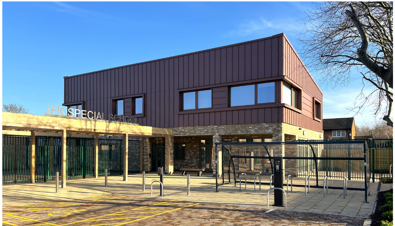
The JFK Special School is part of the Learning in Harmony Multi-Academy Trust, providing specialist education for pupils with additional needs across four sites in Newham. The new extension delivers five purpose-designed classrooms alongside staff accommodation, with a community café creating opportunities for engagement with the local neighbourhood. The project incorporates air source heat pumps and photovoltaic panels to the new extension, delivering a lowenergy-in-use building completed in December 2025.
